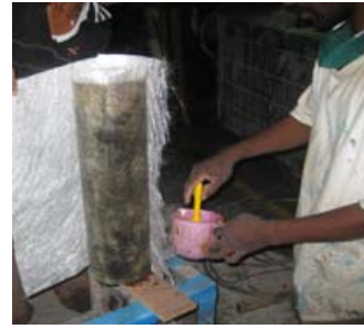
Fig.1 GFRP Wrapping under Progress
